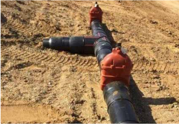
HDPE piping with valves installed ready for installation.
