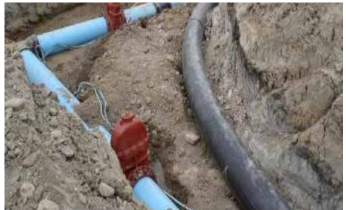
HDPE Pipe (black) vs. traditional PVC piping in blue; Notice how the change of direction is accomplished between the two.
